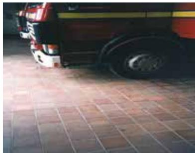
where heavy-duty tiles are used successfully include factory floors, appliance bays in fire stations, loading bays in warehouses and motor vehicle workshops. Heavy duty slip-resistant tiles are also available and should be used in areas which are likely to be wet, trafficked by vehicles, or where increased slip resistance is required.
