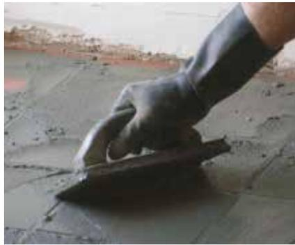
Excess grout should be removed from tile surfaces during grouting using a damp sponge drawn diagonally across the top of the joints. Cleaning off should be undertaken once the grout has hardened sufficiently using a damp cloth or sponge. On no account should sawdust be used for cleaning off as this may enter the joint and reduce its strength. On larger areas rotary scrubbing machines may be used to compact the grout into the joints and facilitate cleaning off.
